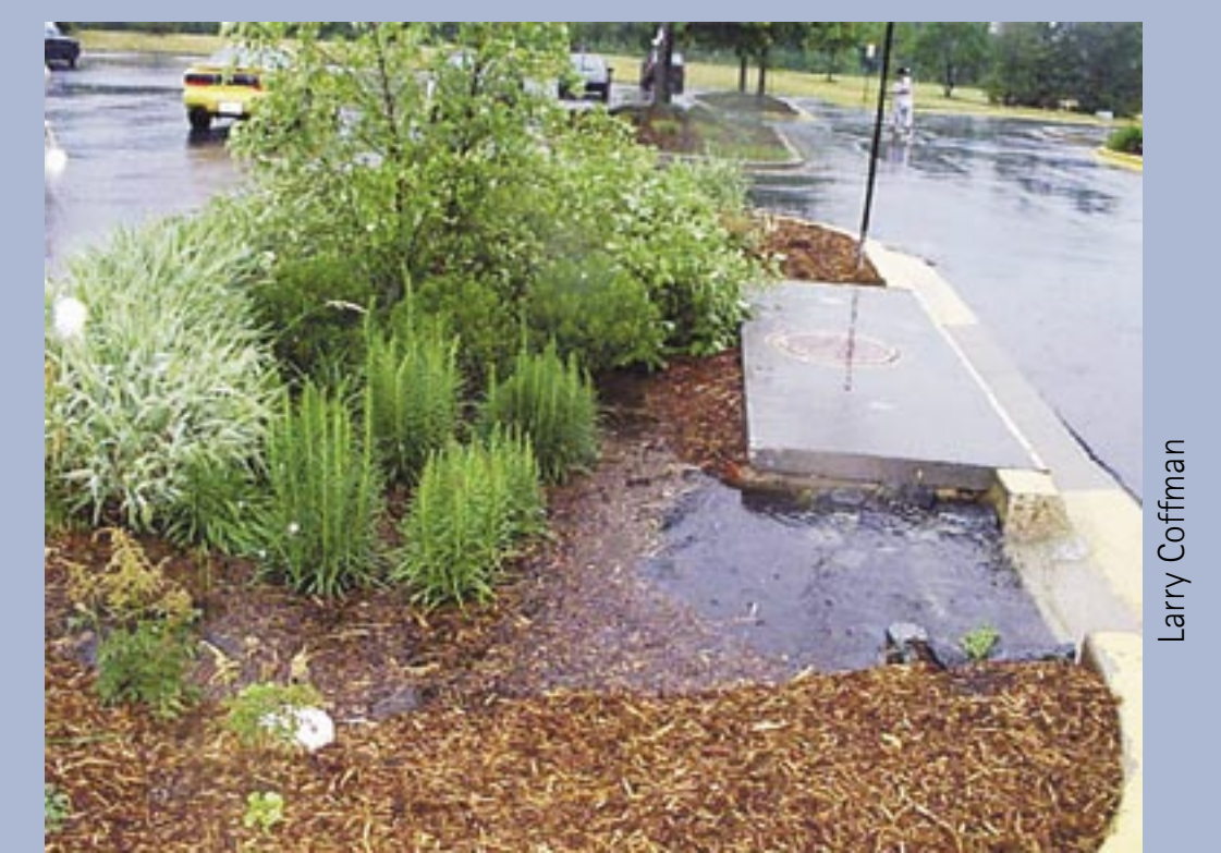
Commercial Bioinfiltration – parking lot detention and infiltration
